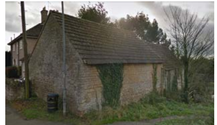
3. Benefield Road - Garage/Outhouse
