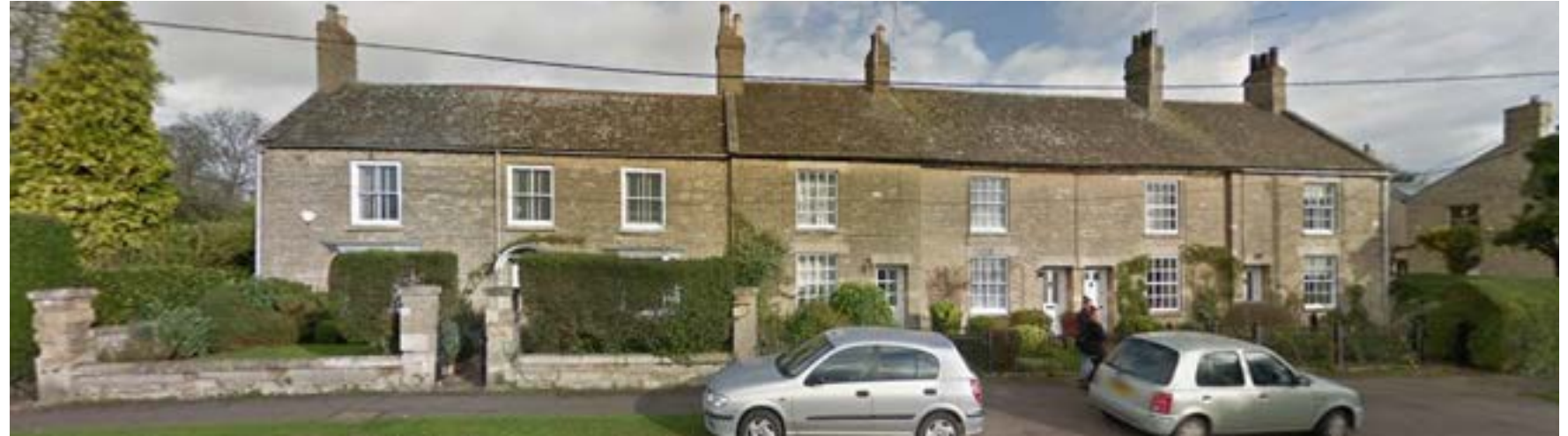
1. Benefield Road - Listed Terrace Houses
